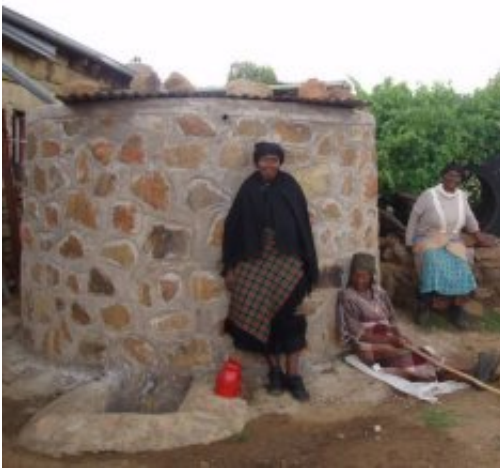
A farmer has roofed her tank with corrugated iron
