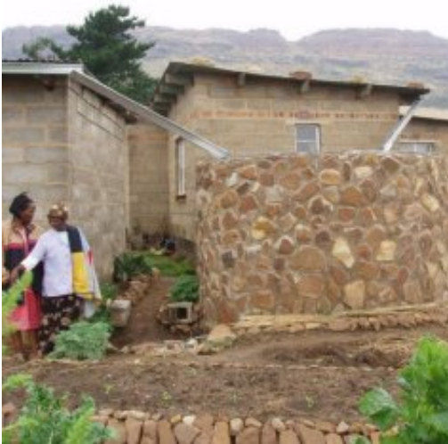
Tank collecting water from two roofs
